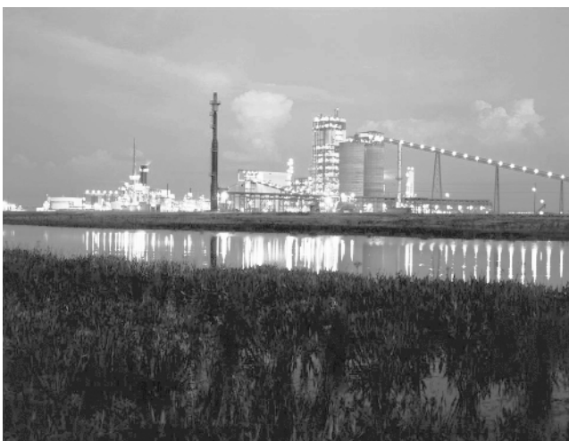
Figure 1.14. Tampa Electric's Polk IGCC Power Station Unit 1. Photo courtesy of Mr. Mark J. Hornick of Tampa Electric.
