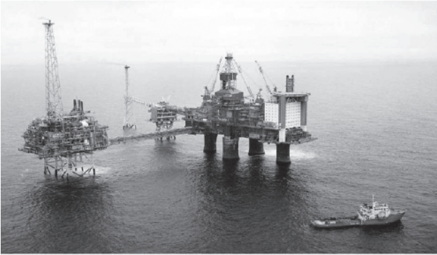
The Sleipner field – \text{CO}_2 Treatment and Injection
