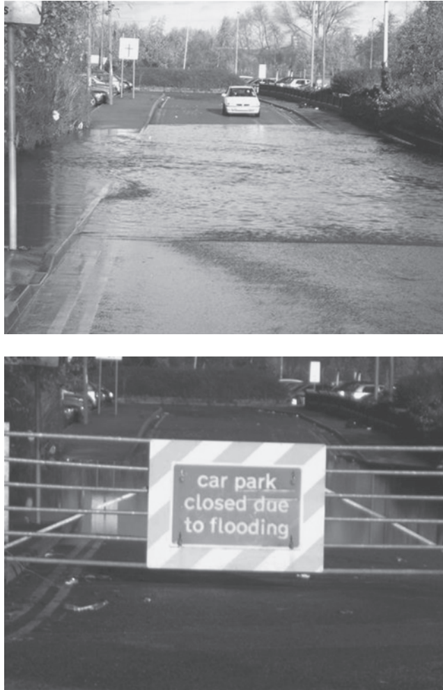
Figure 1.1 An example of a flooded car park where the impermeable asphalt surface is retaining stormwater runoff.
