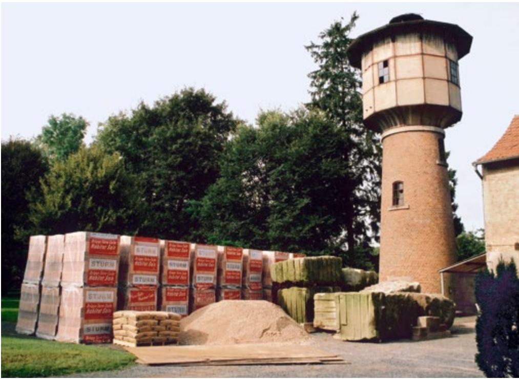
Baumaterial, Wasserturm / Water Tower: Construction Materials, Phalsbourg, 2000.
